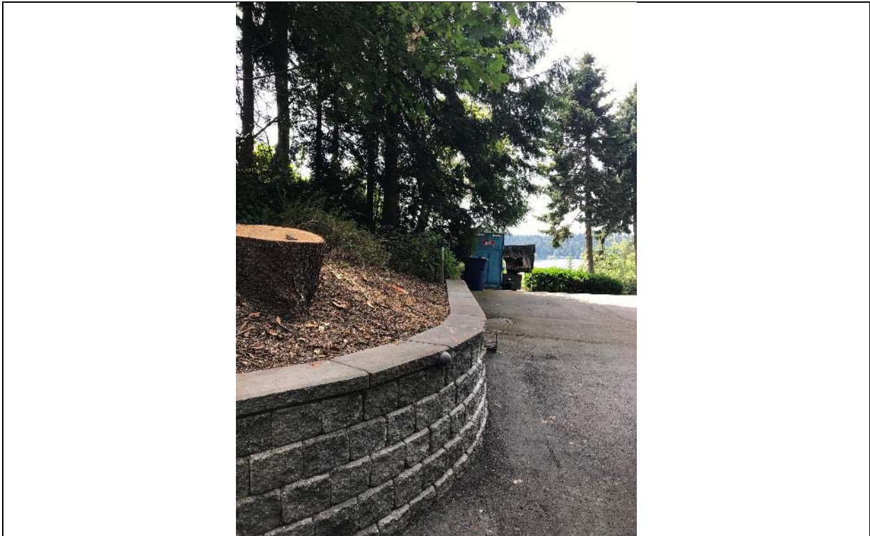
Plate 3. New Redi-Rock gravity modular block wall planned south of existing modular block wall, facing west.
